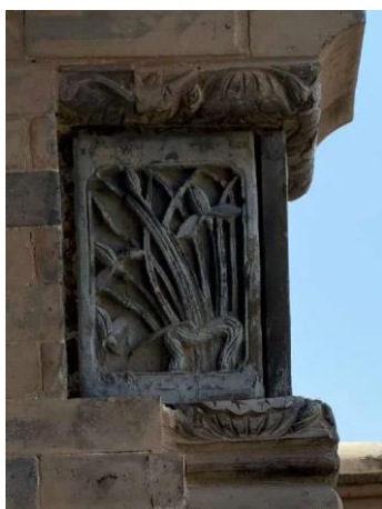
Figure 13. Brick carvings of Baijia Courtyard.
