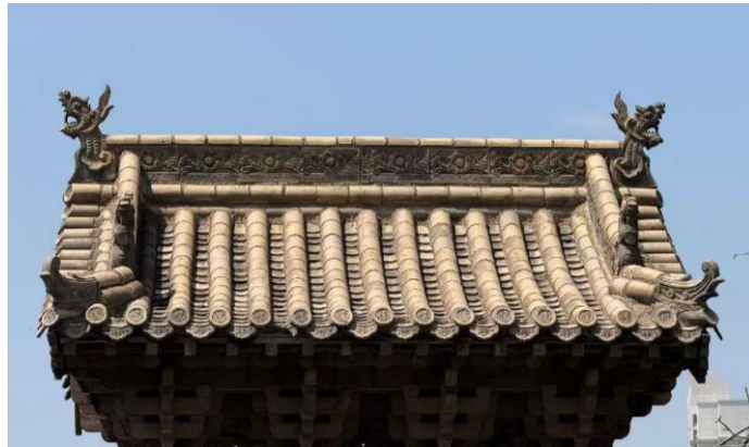
Figure 12. Roof construction of Baijia Courtyard.
