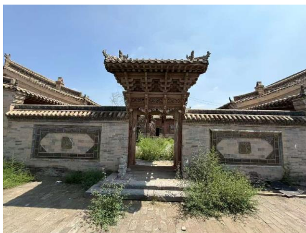
Figure 14. Brick-carved screen wall of Baijia Courtyard.
