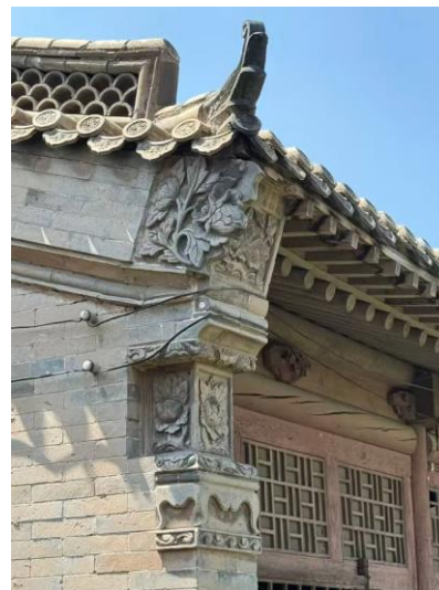
Figures 4. Side view of brick carvings on the gable-end piers of Baijia Courtyard.
