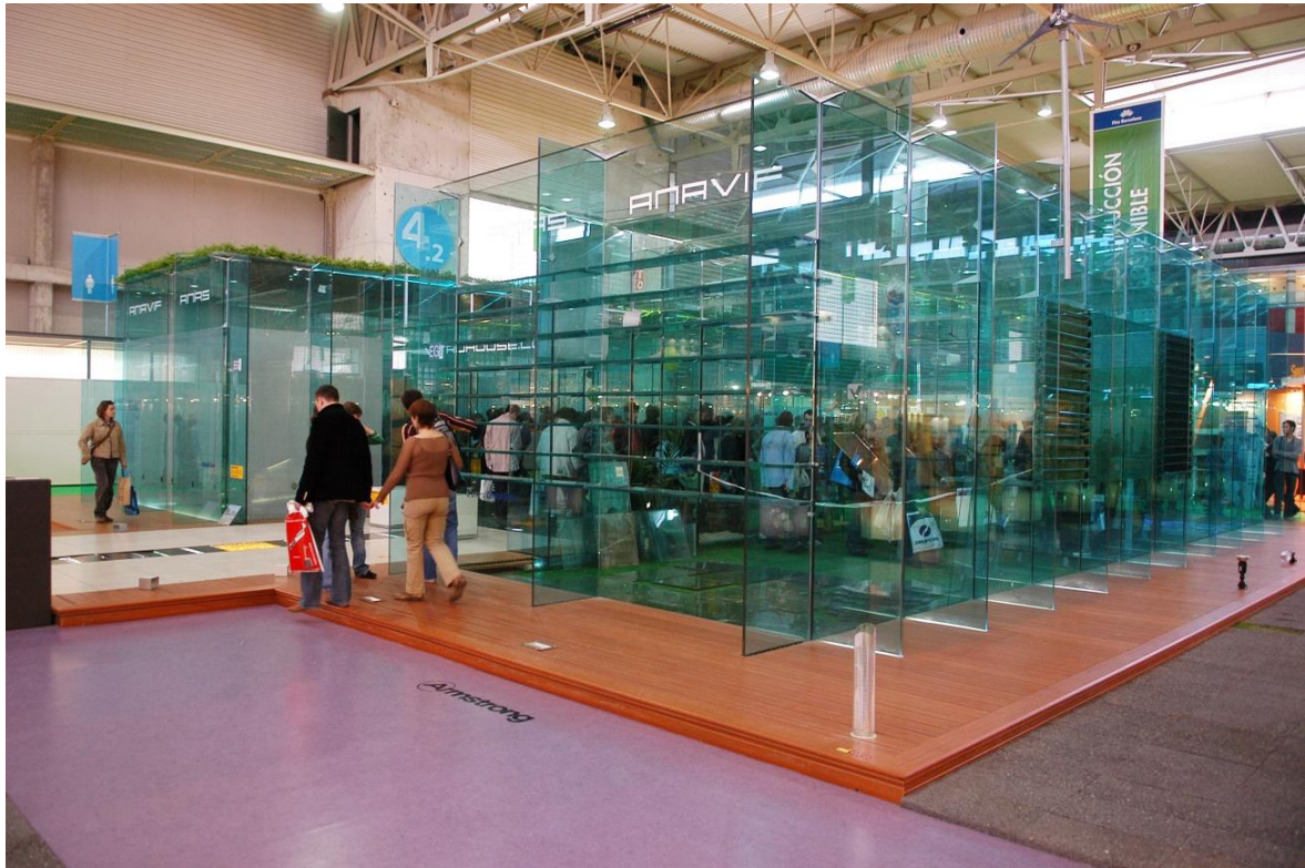
Fig. 9 The right side of Vitrohouse is completely transparent, and thermal insulation is achieved by injecting hot or cold air into the triple skin of the architectural envelope. The air is drawn in from inside the house as it is renovated.
