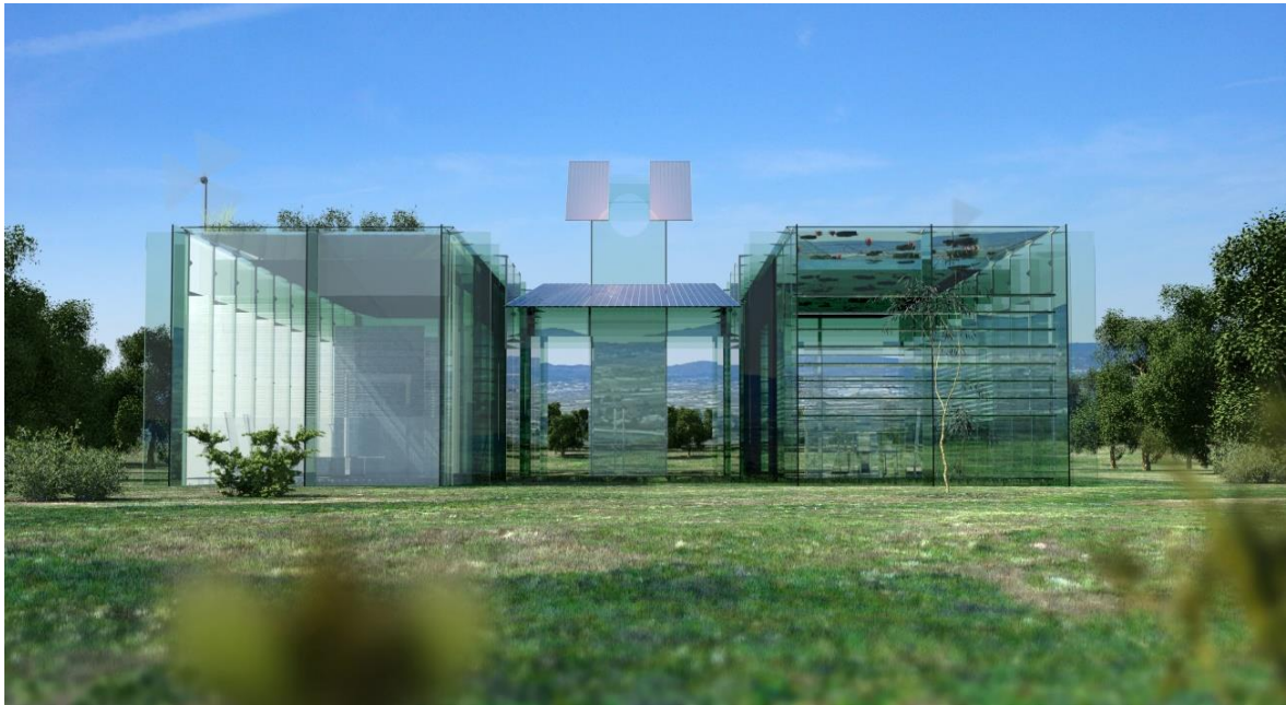
Fig. 4 The central roof of Vitrohouse is composed of two layers of flat glass and integrates solar panels on its exterior, which in turn provide thermal insulation and solar protection to the interior.
