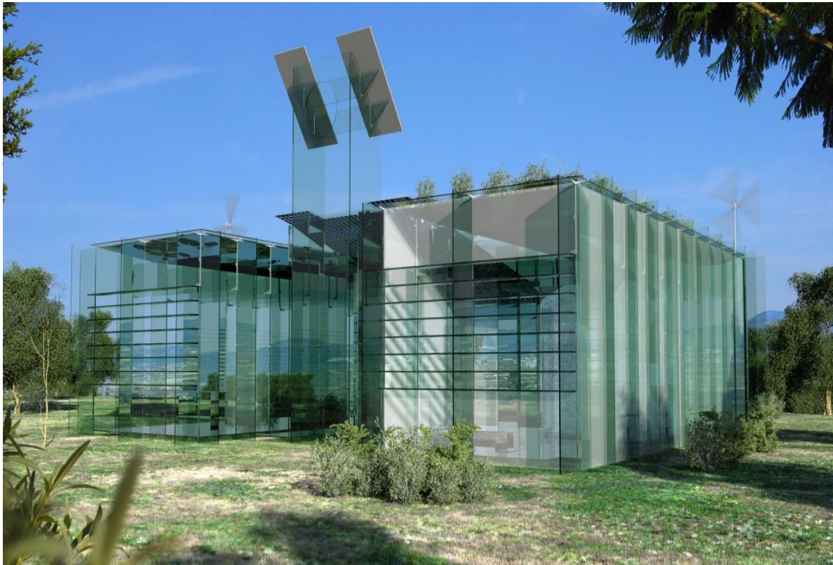
Fig. 2 Vitrohouse is an energy-self-sufficient home that integrates fresh air-capturing chimneys, solar thermal collectors, and photovoltaic solar collectors (project by Luis de Garrido).
