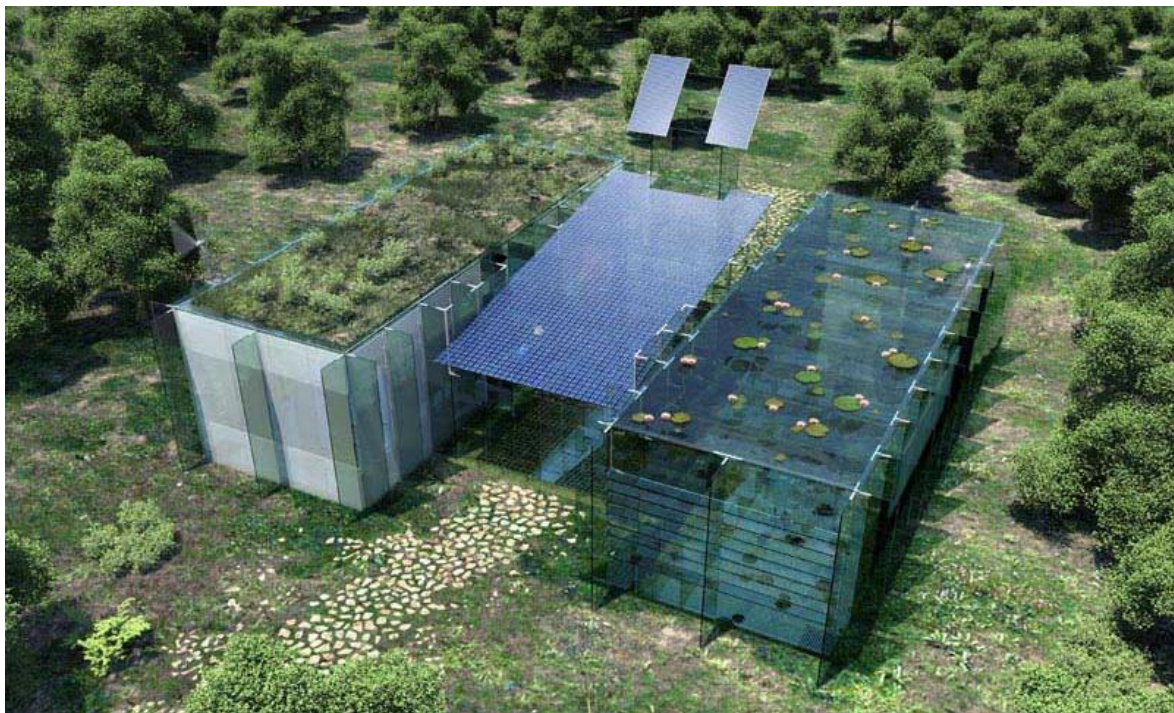
Fig. 1 Vitrohouse was built using only removable components made of flat glass (project by Luis de Garrido).
