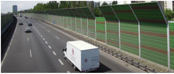
Fig. 1 View of a noise barrier with a height of 8.5 m.
