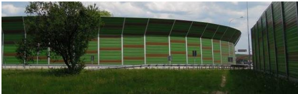
Fig. 2 View of a noise barrier curve in horizontal plane.
