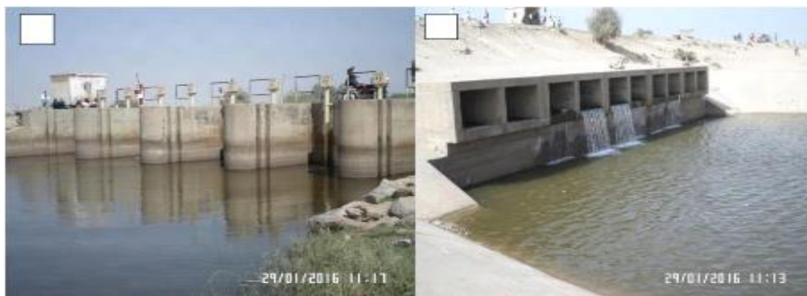
Figure 4. Lake Maga floodgates.
