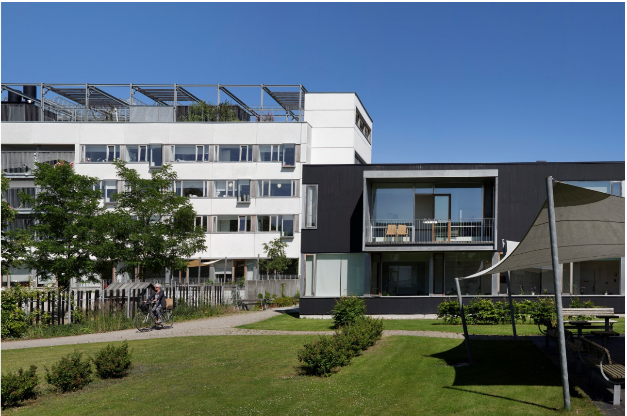
Fig. 10 Buildings and outdoor spaces in Gyldenrisparken after refurbishment.
