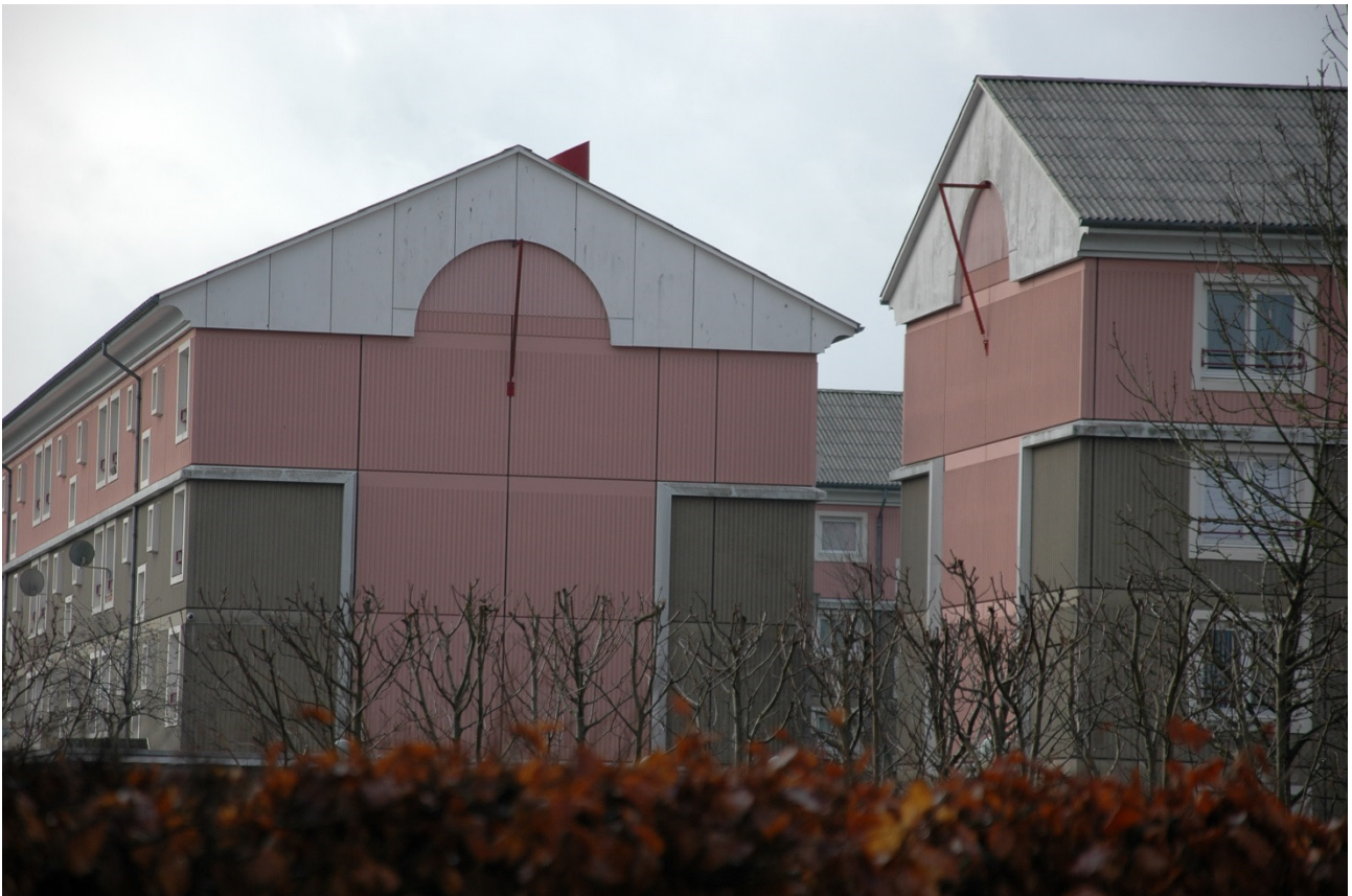
Fig. 2 The first generation of refurbishments in post-war housing areas was developed from 1985-1999. Postmodern colours and ornaments were considered welcome responses to the grey concrete. Roennebaerparken in Roskilde, Denmark. Architect original: Unknown (1968-1970). Architect refurbishment: Mangor & Nagel (1994).
