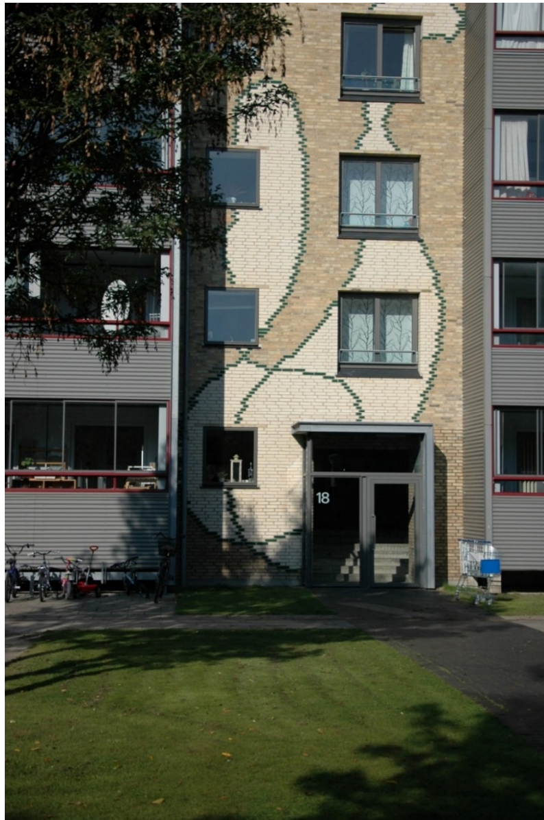
Fig. 3 In the second generation of refurbishment (2000-2009), façades were covered by more traditional materials. Here the original concrete of the façades was hidden away, and artists created organic patterns on the new brick walls. The original architectural expression was erased. Vejleaparken south of Copenhagen, Denmark. Architect original: Tormod Olesen (1970-1974). Architect refurbishment: Domus Architects (2004-2008).
