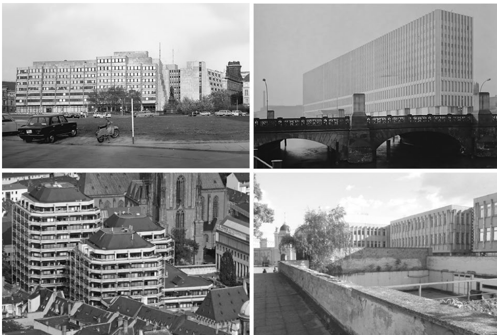
Fig. 3 Demolitions (from top left): Police Headquarters, Dresden; Foreign Ministry, Berlin; Technical Town Hall, Frankfurt a. M.; Teacher Training Institute, Potsdam.
