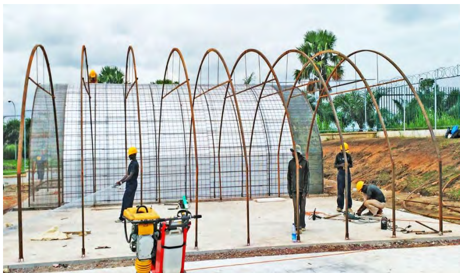
Fig. 6 Putting up of steel arches.
