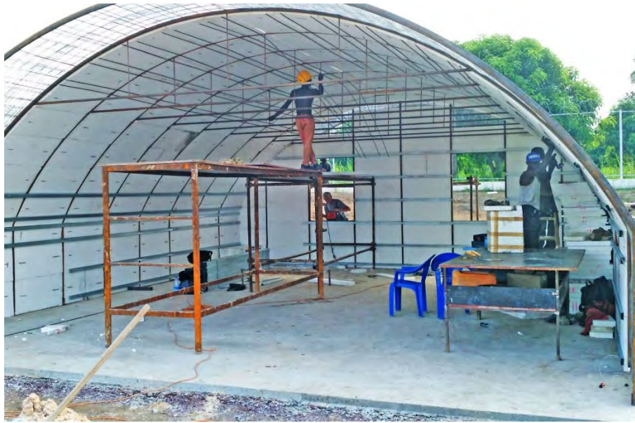
Fig. 10 Installation of polystyrene boards.
