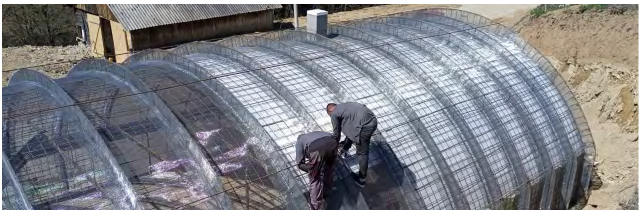
Fig. 28 Placement polystyrene boards.
