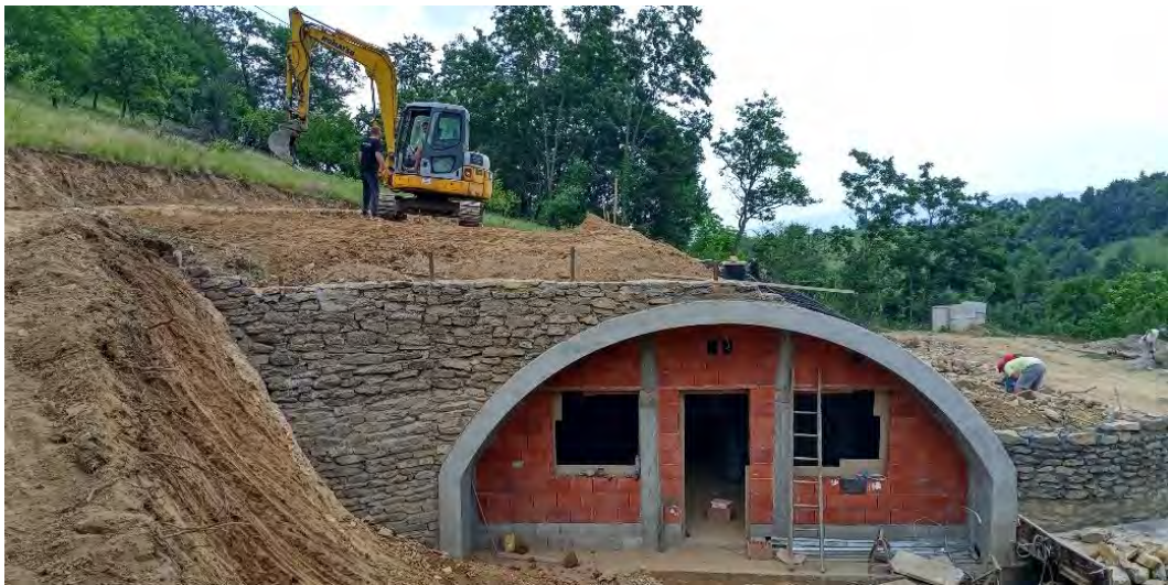
Fig. 30 Covering with soil.
