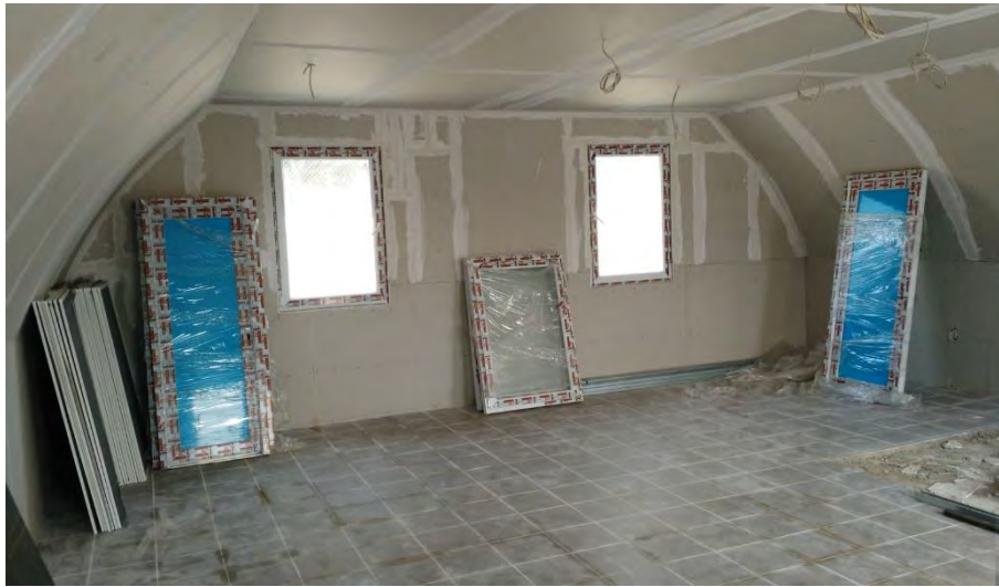
Fig. 15 Installation of plasterboards.
