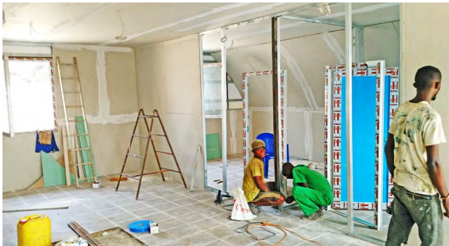
Fig. 15 Installation of plasterboards.
