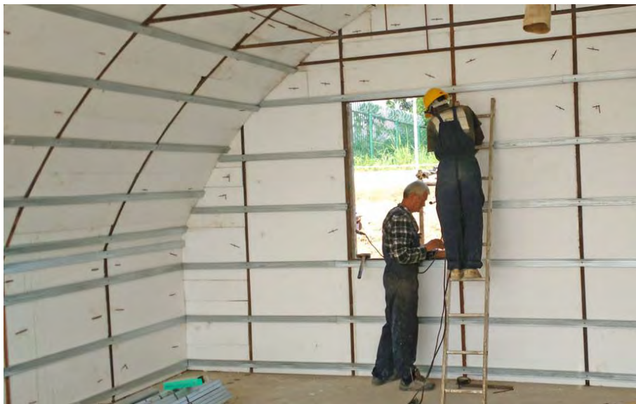
Fig. 13 Installation of plasterboards supports.
