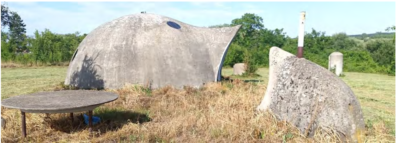
Fig. 34 The first ferrocement object 41 years old.
