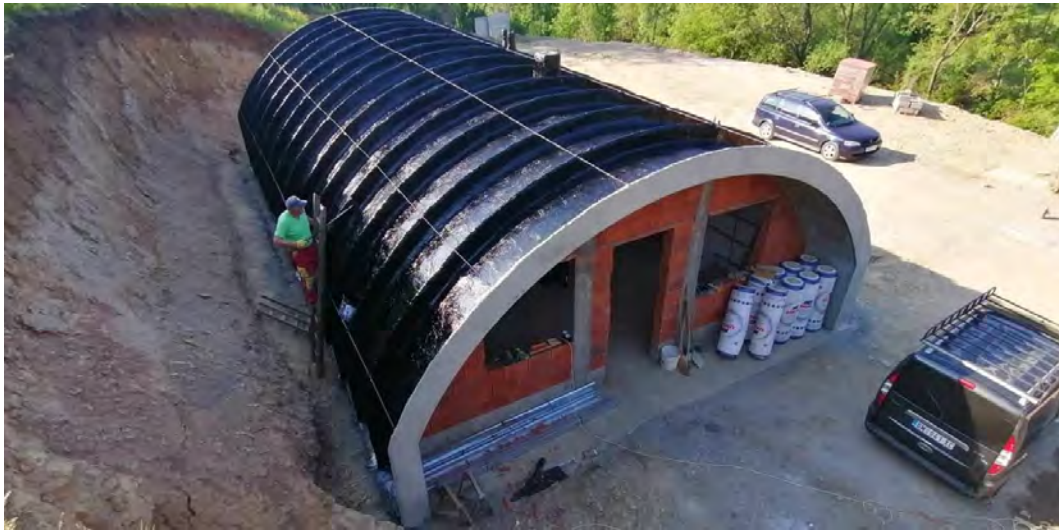
Fig. 29 A waterproofing.
