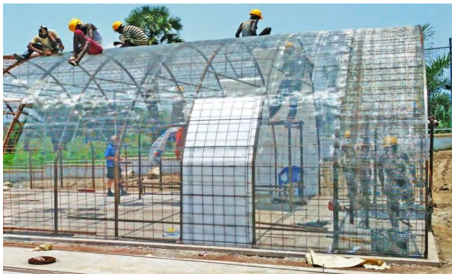
Fig. 9 Putting up galvanized wire mesh.
