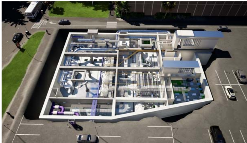
Fig. 3 SWIP AWTF rendering showing treatment plant facilities located below Civic Center parking lot.
