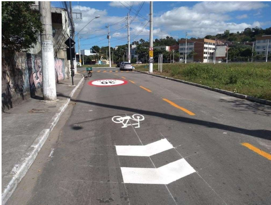
Fig. 1 First route chosen to receive flagged cyclization in Goiabeiras.
