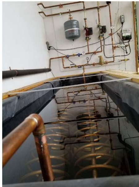
Fig. 11 Thermal battery, heat exchanger and the system manifold.
