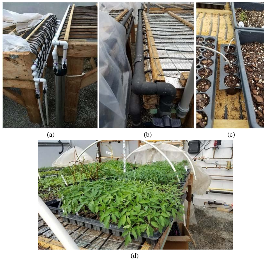
Fig. 4 Heat distribution with root zone heating (RZH) system: (a) header pipes and ethylene propylene diene monomer (EPDM) tubing on benches; (b) polyvinyl chloride (PVC) painted with latex for ultraviolet (UV) protection; (c) temperature sensor in the germination table; (d) plants on heated bench.
