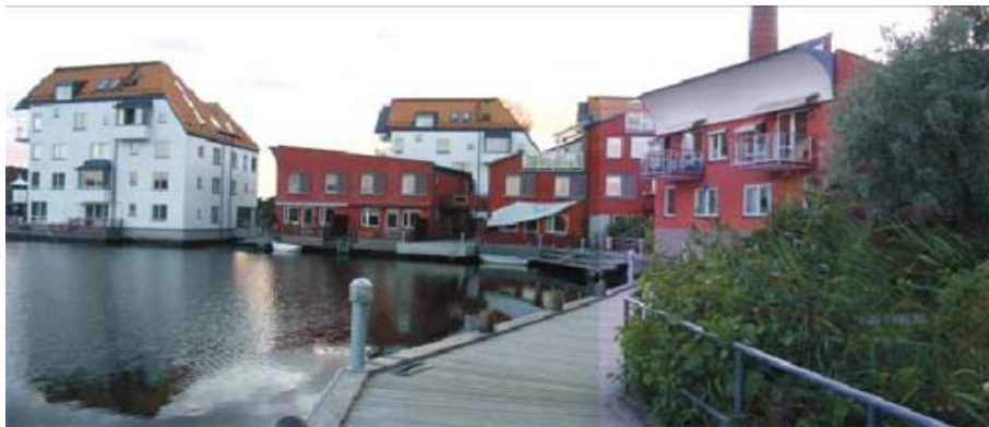
Fig. 5 Lakefront surrounded by the wooden pathway and diverse building forms.
