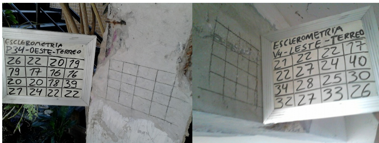
Fig. 3 Sclerometry test detail.
