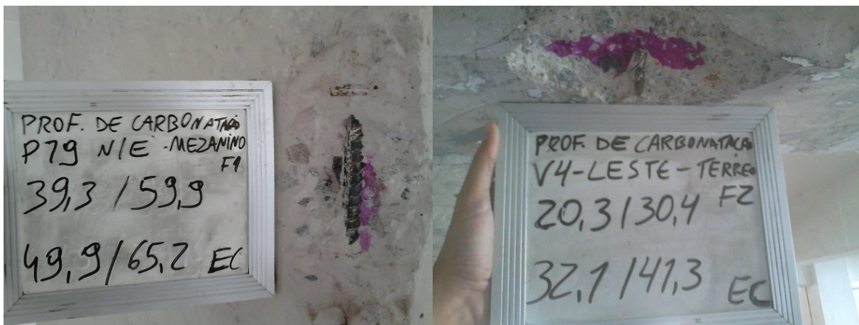
Fig. 2 Concrete carbonation/cover thickness test.
