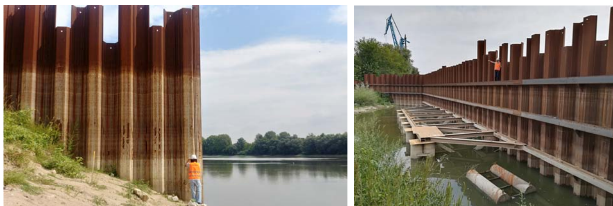
Fig. 3 Cofferdam from steel sheet piles GU 22N, one can observe the variation of the water levels.
