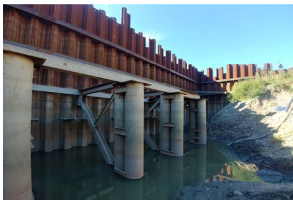
Fig. 3 Cofferdam from steel sheet piles GU 22N, one can observe the variation of the water levels.
