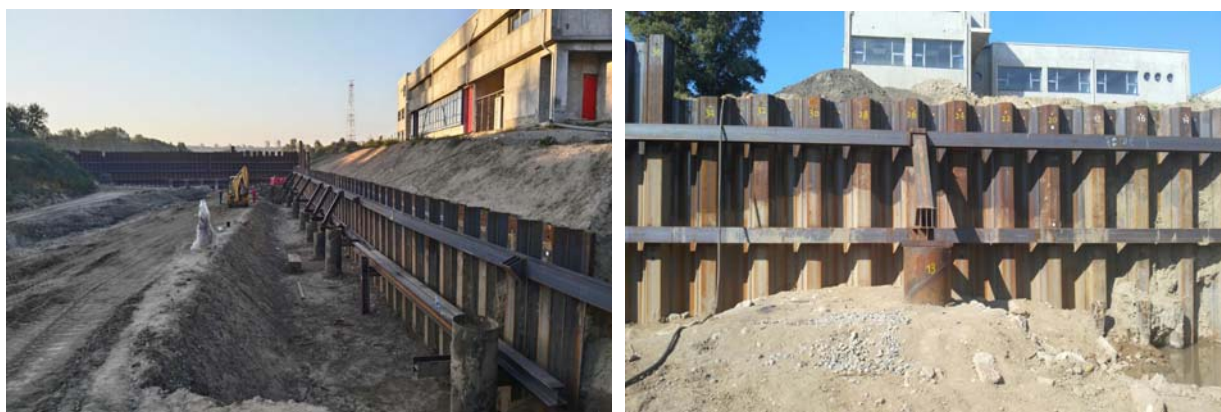
Fig. 13 Retaining structure on the side of the AFDJ neighborhood.
