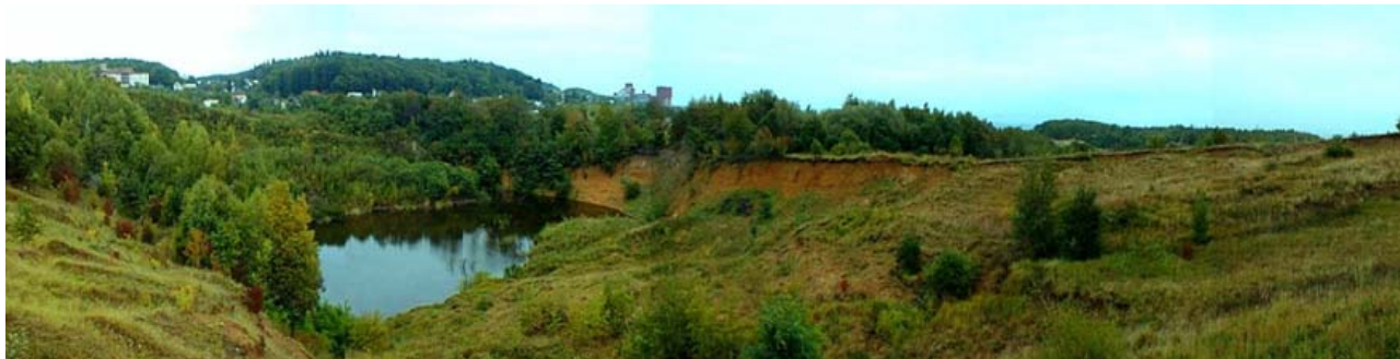
Fig. 5 The Subsidence over the magnesite mine Košice-Bankov, panoramic view: spring 2002 [19-21].
