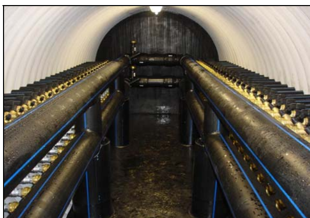
Fig. 8 The new type of field manifold, that was first applied at IKEA Helsingborg 2010.
