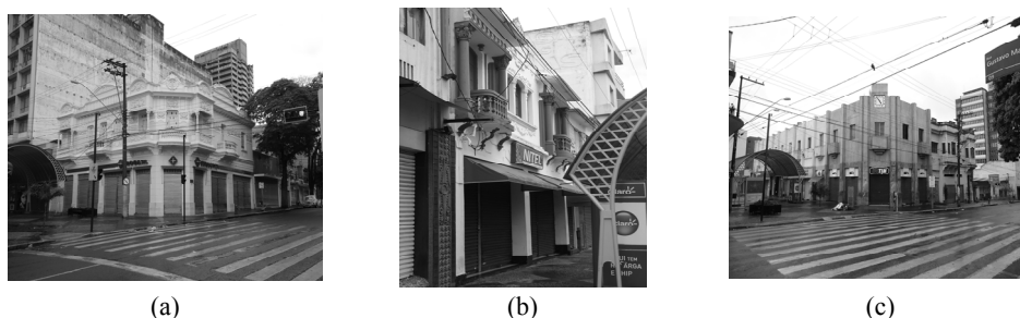
Fig. 3 Buildings listed by CODEPAC: (a) Palace Pagani; (b) Older Commercial House; (c) Lusitana House.
