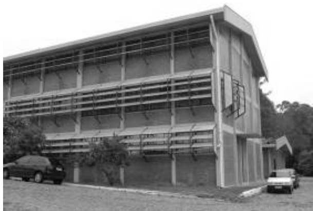
Fig. 1 G1 building—north facade.
