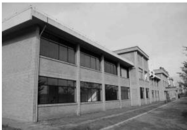
Fig. 2 L1 building—north facade.
