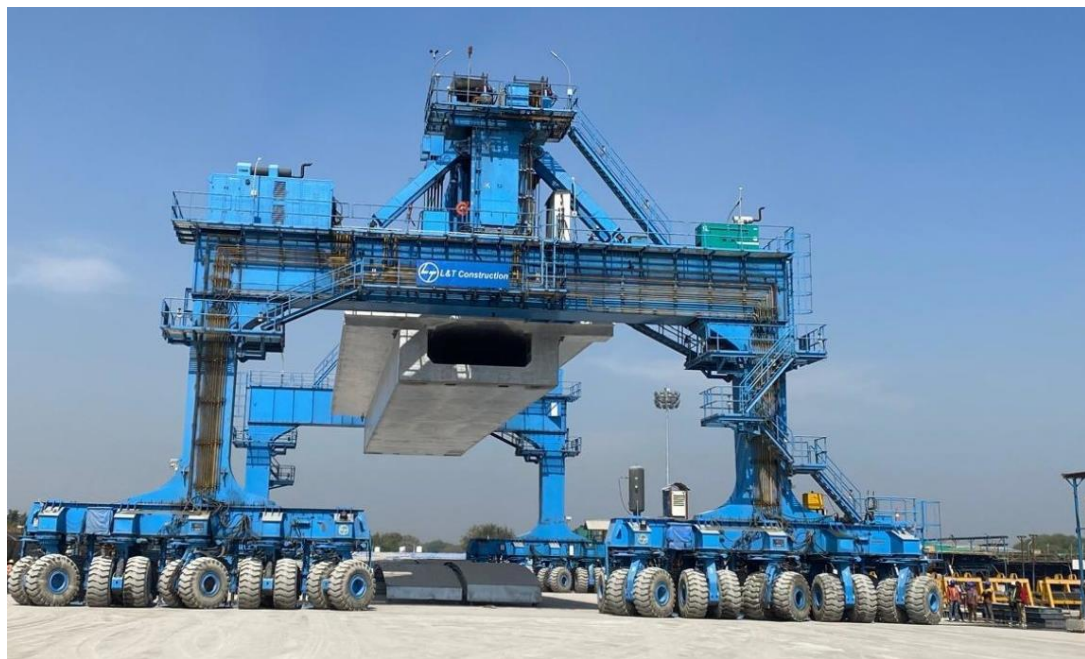
Fig. 11 Straddle carrier lifting and shifting the FSLM girder.
