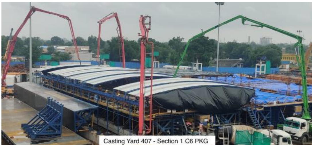
Fig. 10 Casting in progress in rainfall season.
