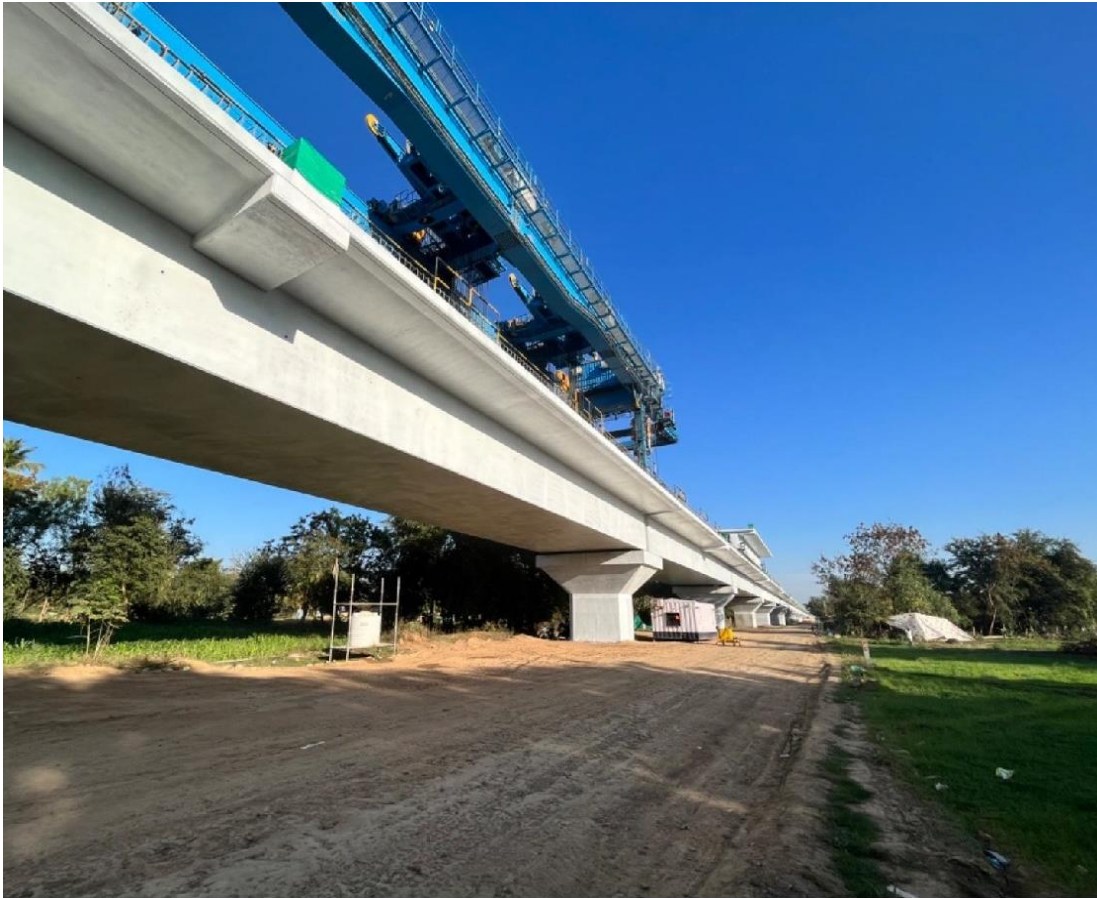
Fig. 2 Successfully launched FSLM girders.
