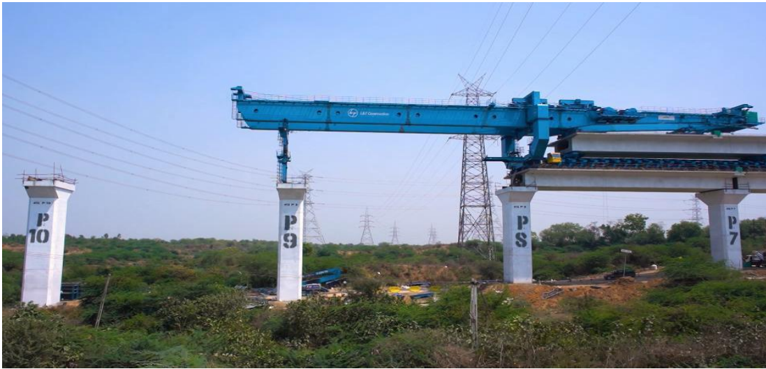
Fig. 16 Launching gantry after GT entry.
