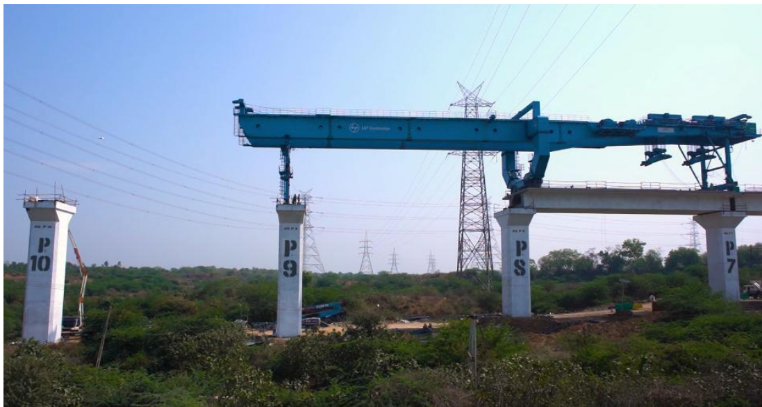
Fig. 15 Launching gantry after auto-launching.
