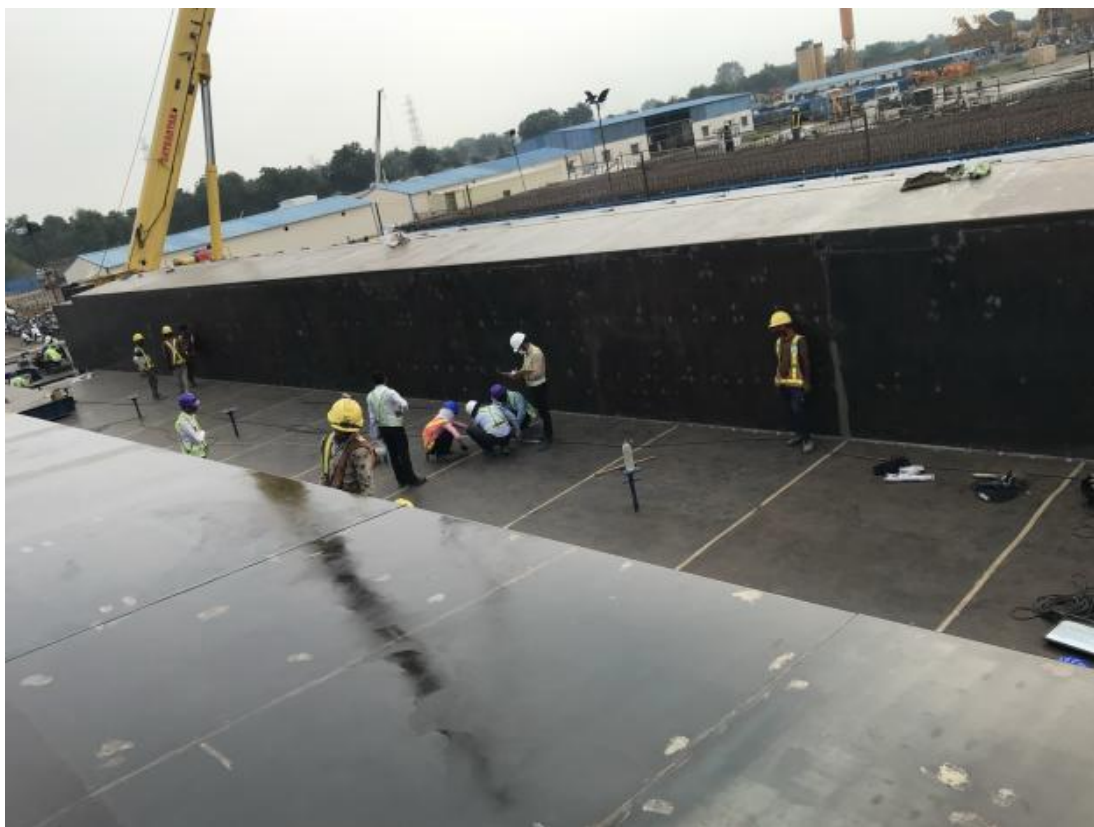
Fig. 8 Outer shuttering survey checks.
