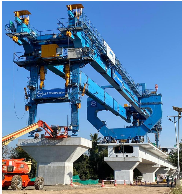
Fig. 14 Launching gantry getting ready for new FSLM girder erection.
