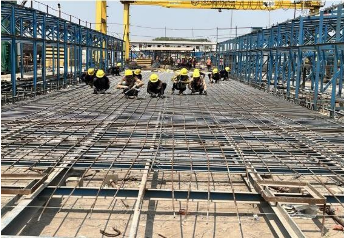
Fig. 5 Reinforcement cage fabrication.
