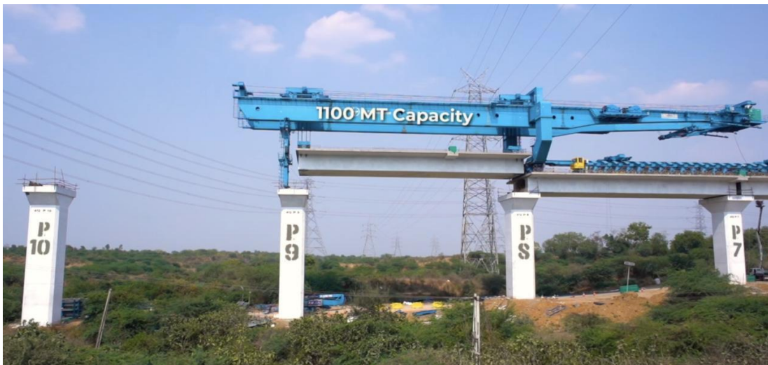
Fig. 18 Launching gantry during FSLM girder lowering.
