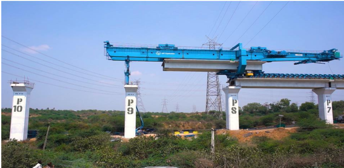
Fig. 17 Launching gantry during girder lifting.
