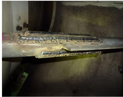
Fig. 25 Welding is complete.
