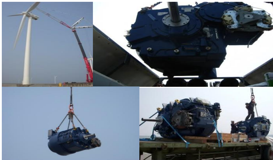
Fig. 14 Wind turbine gearbox hanging project.
