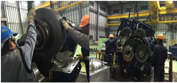
Fig. 15 Gearbox maintenance project.
