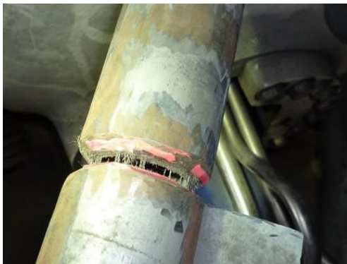
Fig. 22 Weld preparation.
