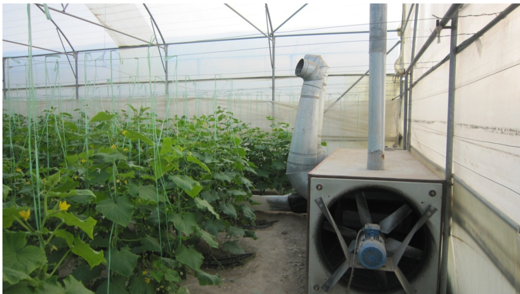
Fig. 2 Greenhouse with gas heater system.
