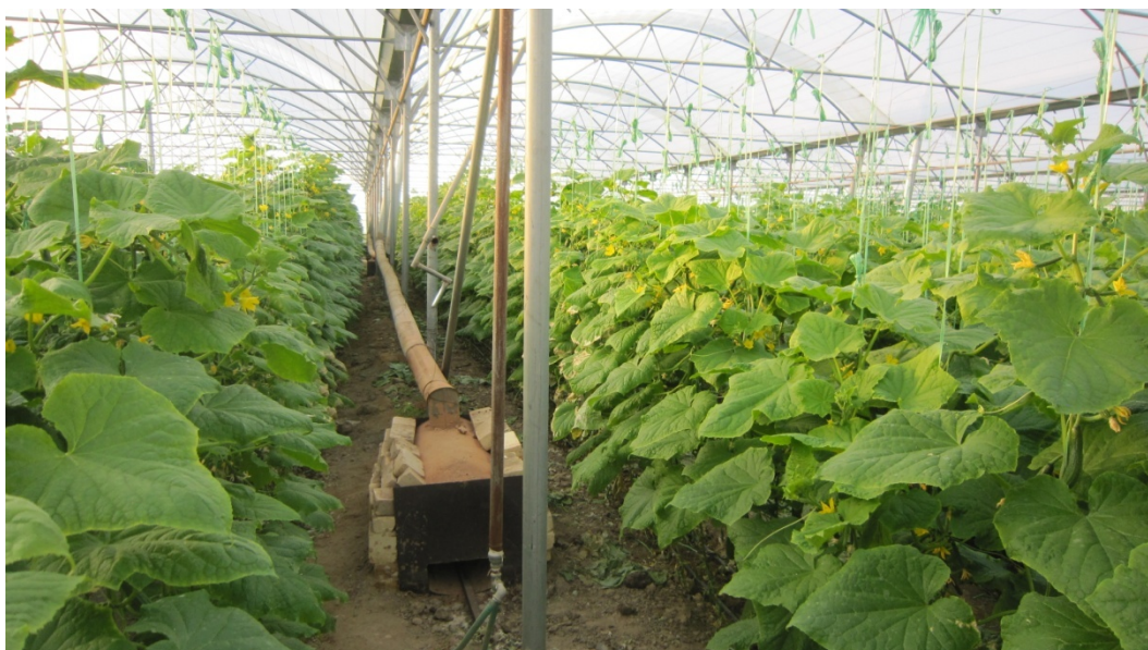
Fig. 3 Greenhouse with traditional furnace system.
