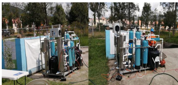
Fig. 5 Wastewater treatment double advance oxidation plant.
