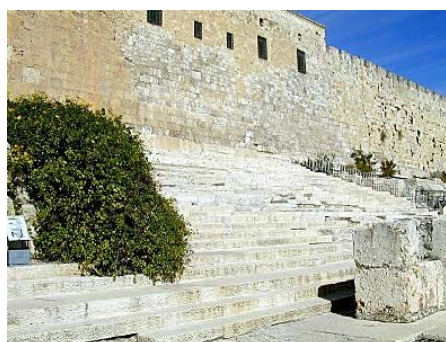
Figure 11. General view of steps. 20
