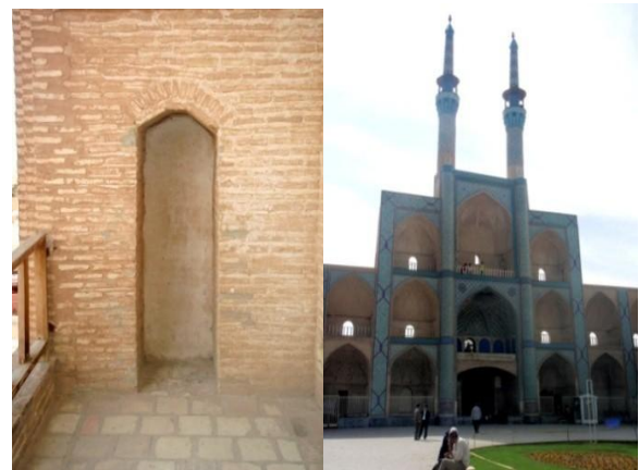
Fig. 12 Voids in walls which allow the lightening of structure.
