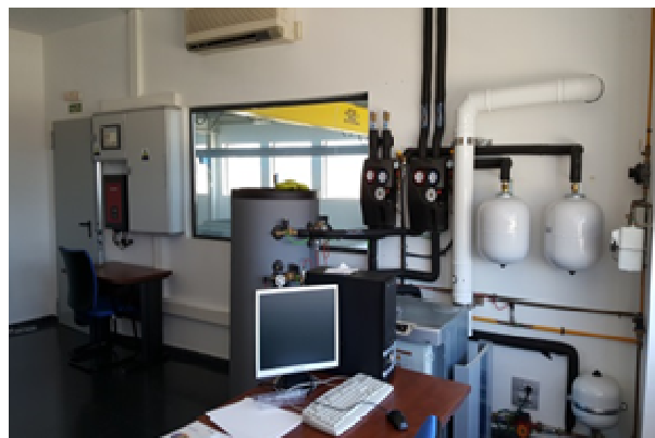
Fig. 1 Cogeneration laboratory facilities.
