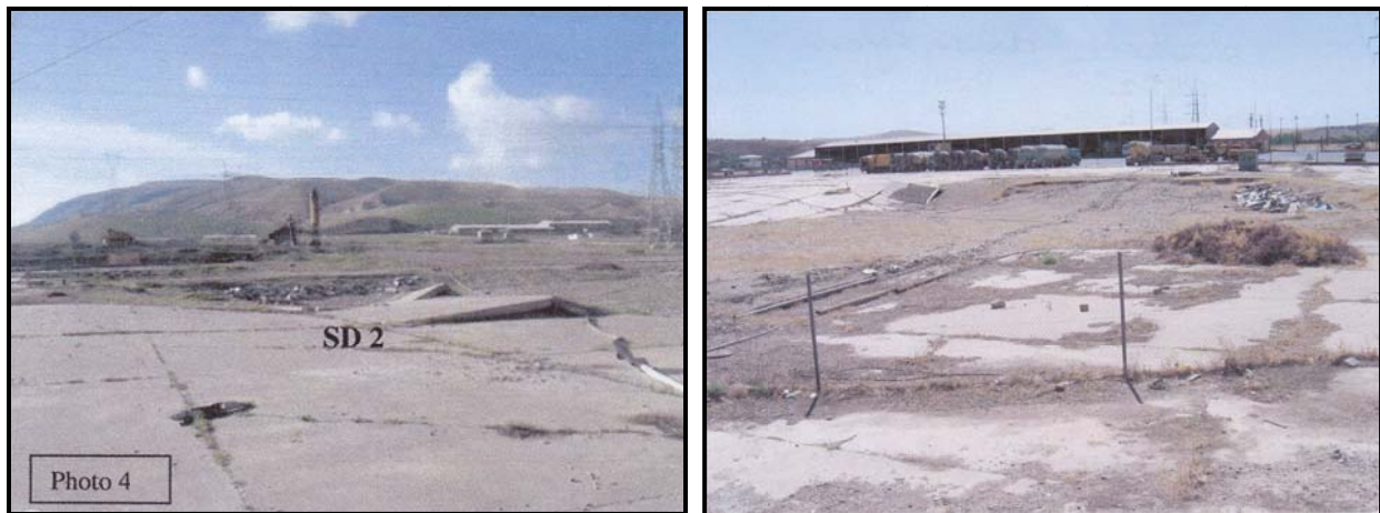
Fig. 20 Two views of sinkhole SD2 at the initial stage and final stages of development [9].
