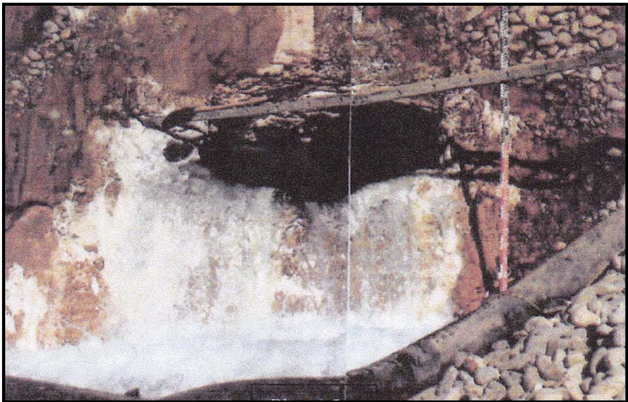
Fig. 16 The flow (360/sec) from underground aquifer into the intake/tailrace tunnel of the pump storage scheme originating from Wadi Der Malih aquifer [9].
