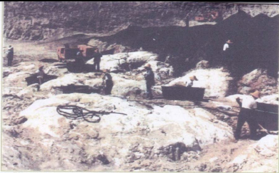
Photo 1. Chute area of the spillway, top of GB3 layer; subrounded boulders of gypsum/anhydrite and brecciated marls.
