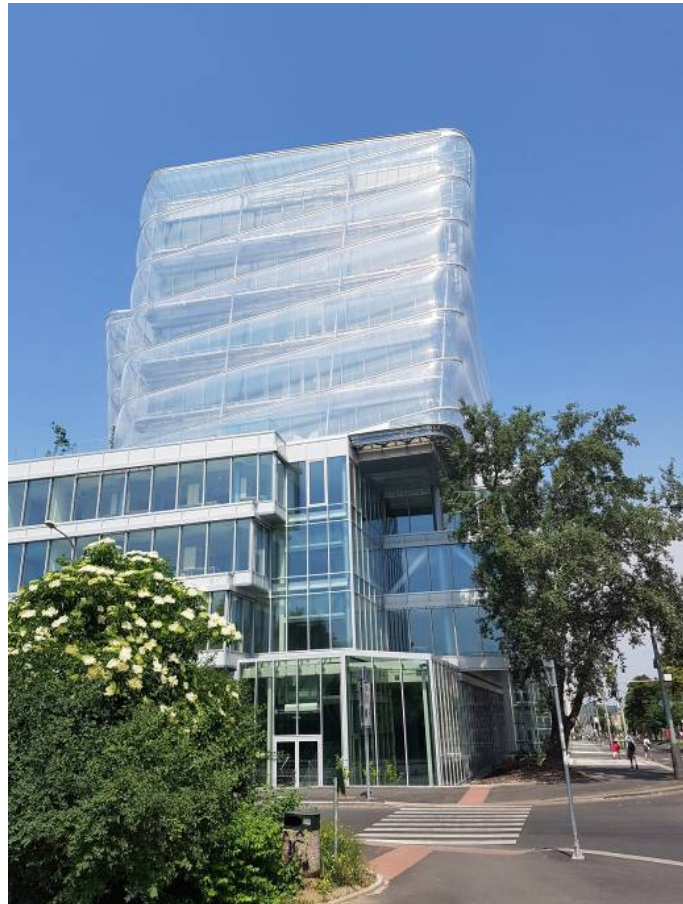
Fig. 1 Double skin façade using ETFE membrane as a solar collector.
