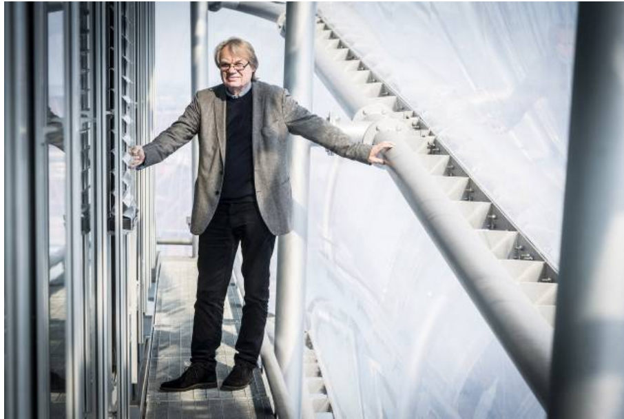
Fig. 7 Space between triple glazing and membrane ETFE, horizontal blinds fixed to mullions on the left. Catwalk is used for maintenance [1].
