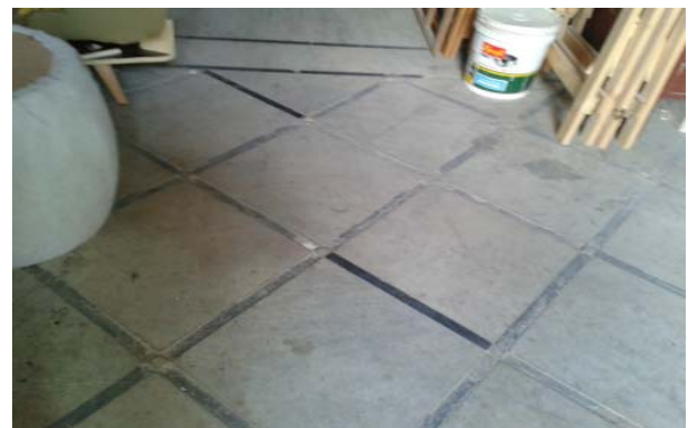
Fig. 21 Poured lime cement tile used in late Ottoman period in Bchara el-Khoury mansion (idem).
