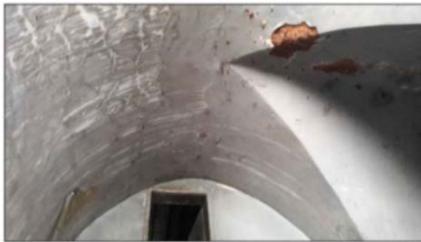
Fig. 18 The arched vaulted floor in kaaki house (idem).
