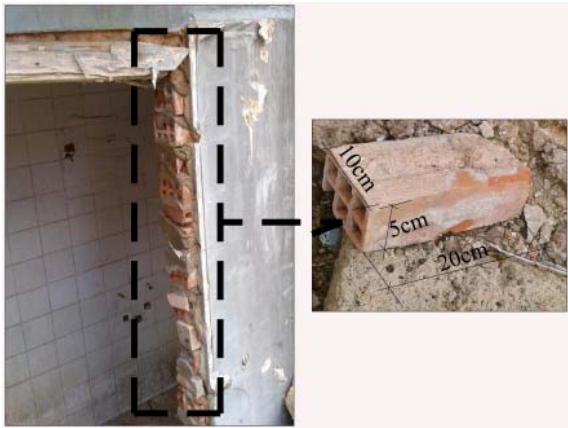
Fig. 25 Showing the brick construction in kitchen and toilet area in Kaaki building (idem).
