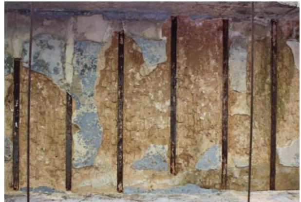
Fig. 4 Jack arch slab at the ground floor.
