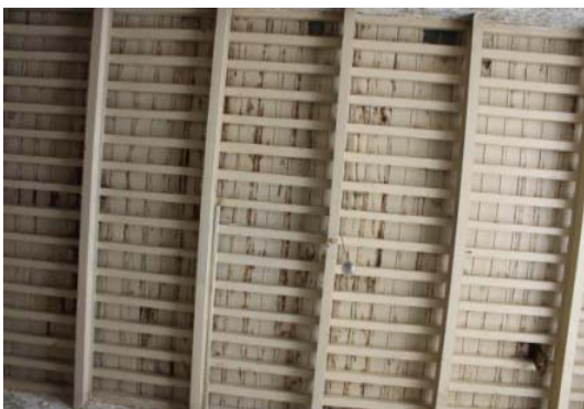
Fig. 15 Timber cut beam in the central hall at first floor (idem).
