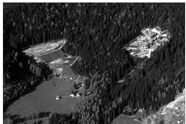
Fig. 4 The two Stava tailings dams and the Prestavèl mine facilities (October 1981).
