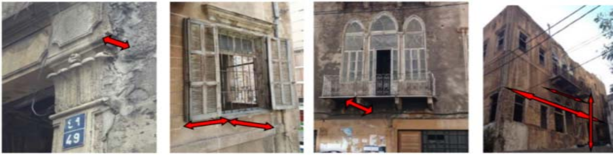
Fig. 5 An example of props, projections and cantilevers in three buildings (Hammoud J. 2016).
