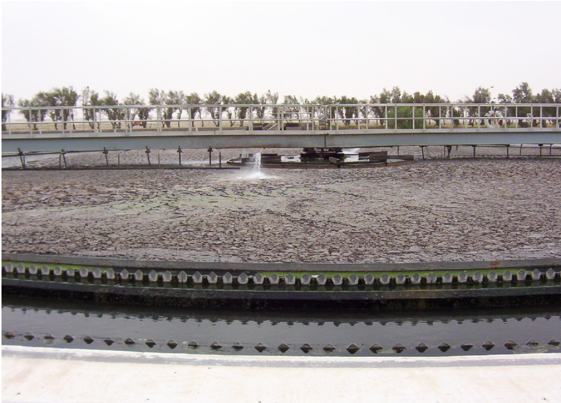
Fig. 2 Floating sludge in clarifier.
