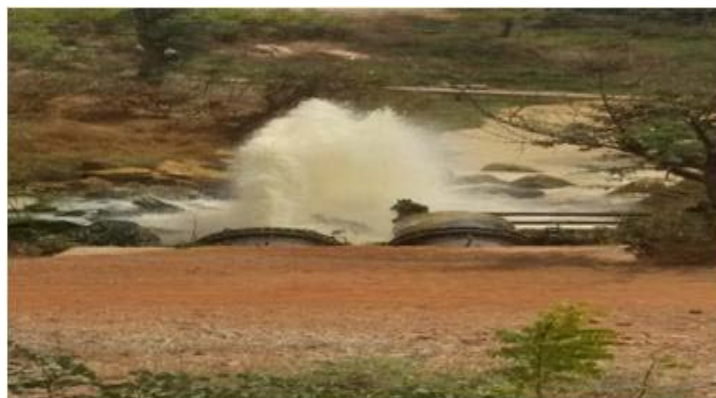
Fig. 1 Gari dam penstock discharge pipe.
