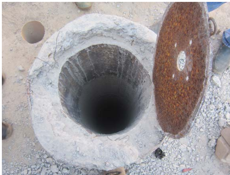
Fig. 3 View of the well used for the investigation of flow velocities in groundwaters.
