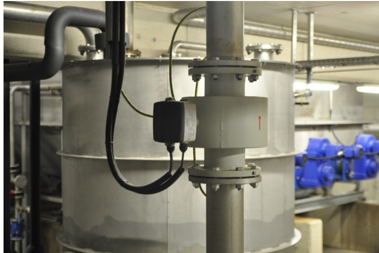
Fig. 2 Reliable even under harshest conditions and high concentrations of impurities: the Transmag 2 flowmeters in the IKB handle up to 40 m 3 an hour.
