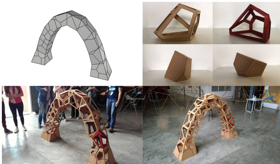
Fig. 3 The digital model, some separate parts, and the finished arch in a 1/2 scale.
