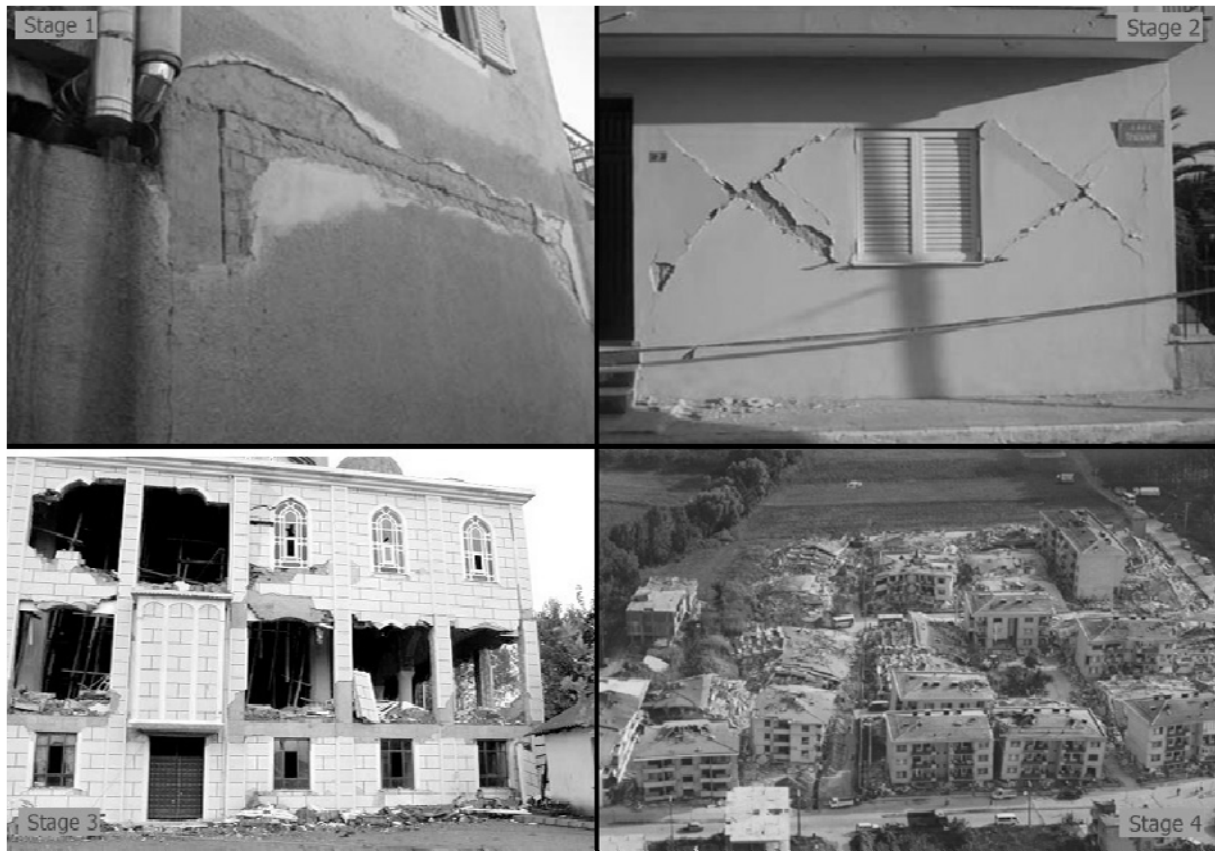
Fig. 1 Stages of infill wall failure on RC structures (from small cracks up till total structural collapse).
