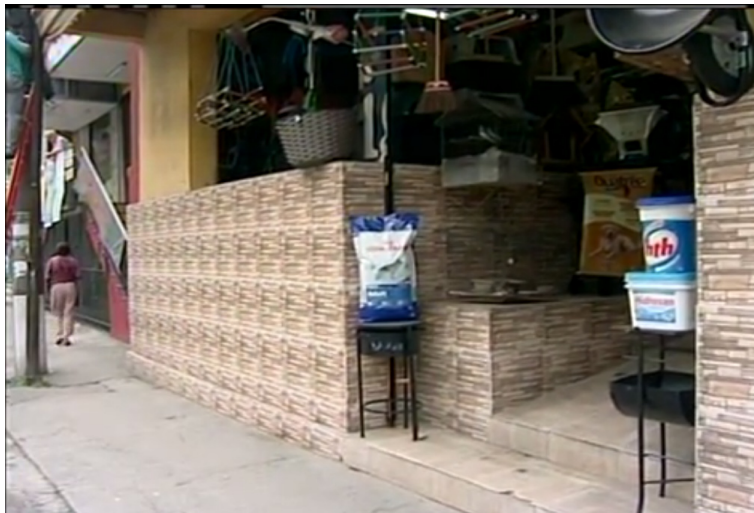
Fig. 6 Shop front flood barrier wall 2 m high [31].
