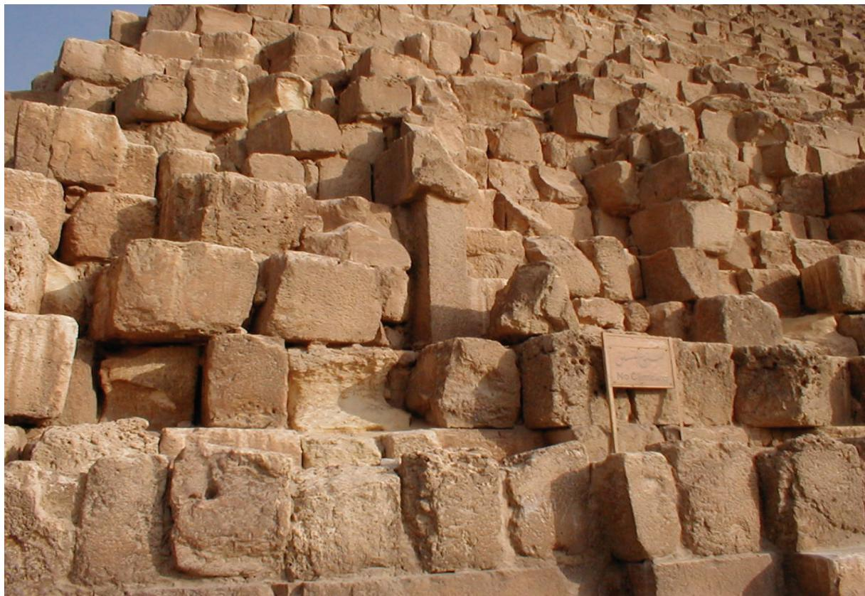
**Fig. 4** The photo presents the north-western corner of the Great Pyramid at Giza, from its western wall. Blocks are arranged irregular, not all spaces between the blocks are filled with mortar (Photo by K. Solek).
