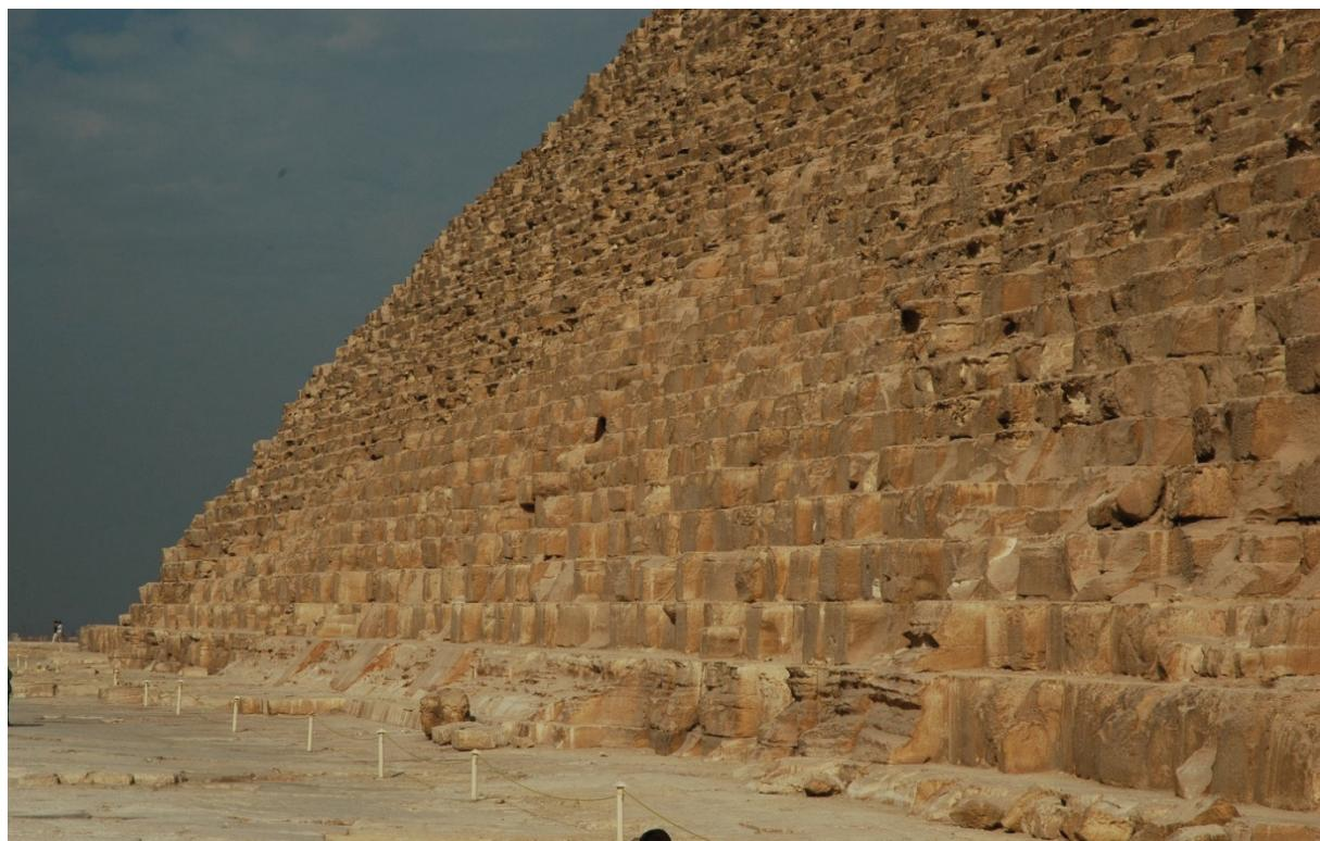
Fig. 13 Western wall of the Great Pyramid at Giza. Strongly eroded casing blocks from the 1st layer and one side of  $\alpha$  triangle are visible. The triangle in the western wall is topped with a single stone. It is located in the 19th layer of blocks, 16 m 65 cm high (Photograph by the author).
