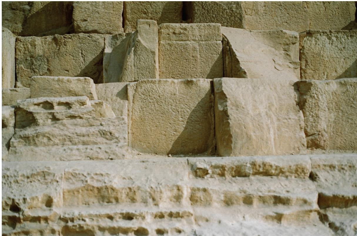
**Fig. 5** In the picture we can see the central part of the western wall of the Great Pyramid at Giza. In the foreground eroded casing blocks are visible. They were fitted in such a detailed way that it is difficult to see the joints between them. The blocks of the 2nd layer of the pyramid are precisely fitted, and the space between them is filled with mortar (Photo K. Solek).
