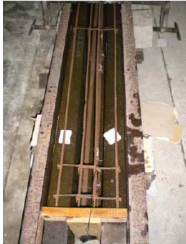
(b) Cages inside mould before casting.
