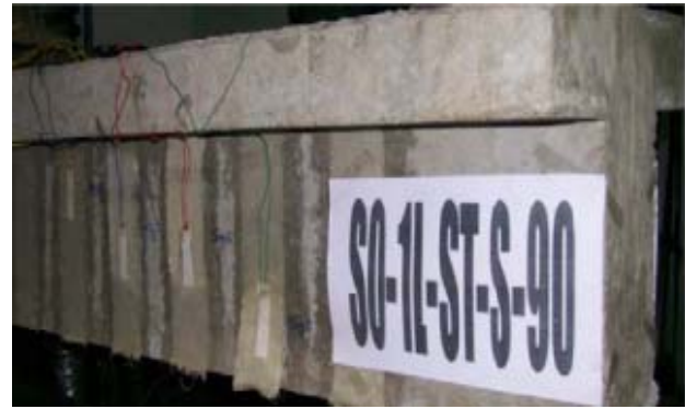
(b) Debonding failure
