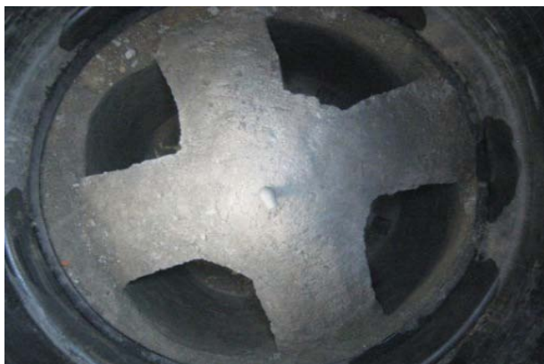
Fig. 3 Pyramid shaped stand on the conical structure supporting gas outlet pipe.
