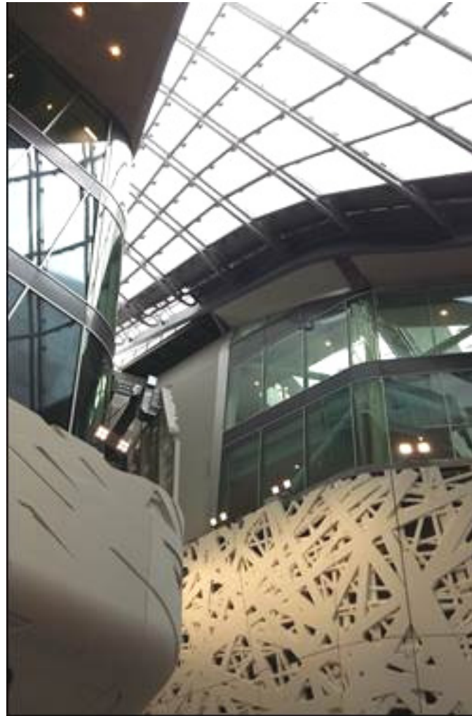
Fig. 11 Palazzo Italia, foyer, roof detail and fiber cement panels.
