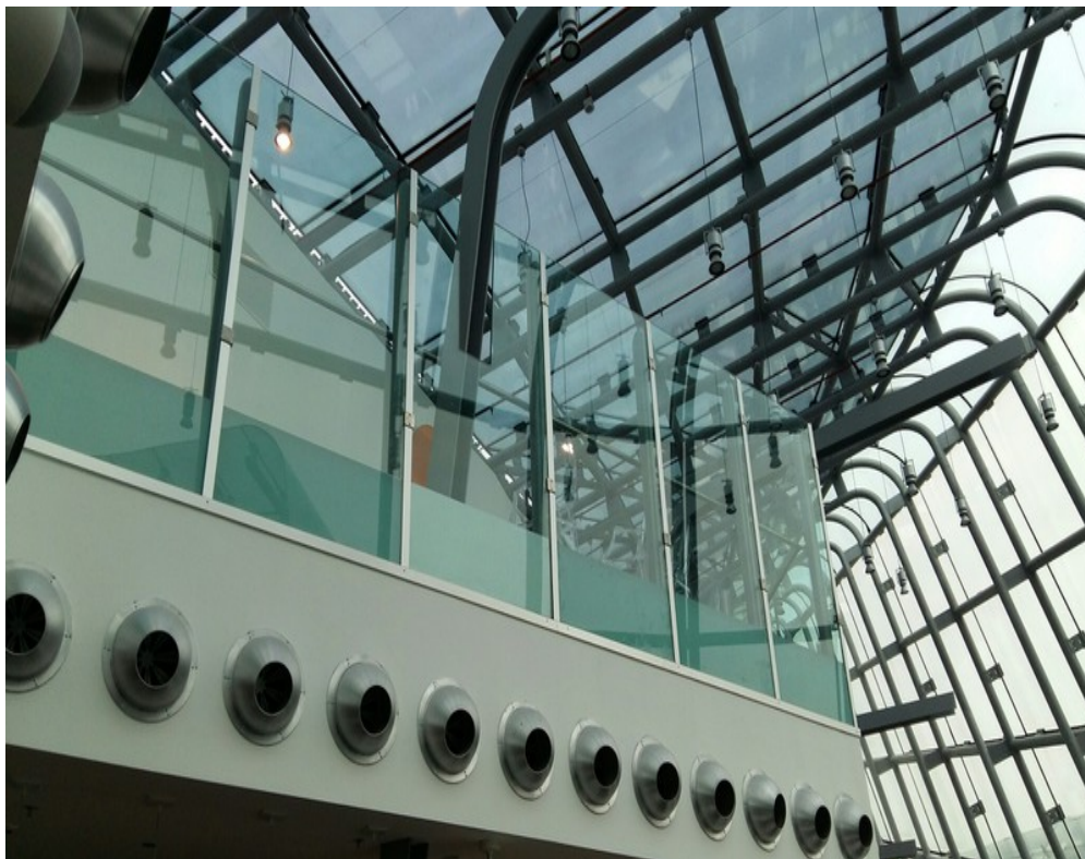
Fig. 9 Palazzo Italia, restaurants space, photovoltaic glass roof.
