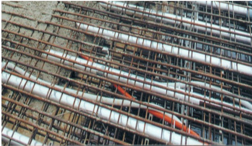
Fig. 4 Tubular systems laid in the reinforcement of the floors with concrete casting.
