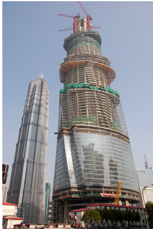
Fig. 3 Shanghai tower of Gensler architects, high 632 m, double skin curtain wall, green technologies with about 200 wind turbines (the highest in the world), top of the tower, which produce about 10% of total electricity.
