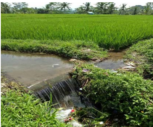
Fig. 3 Damaged irrigation canal.
