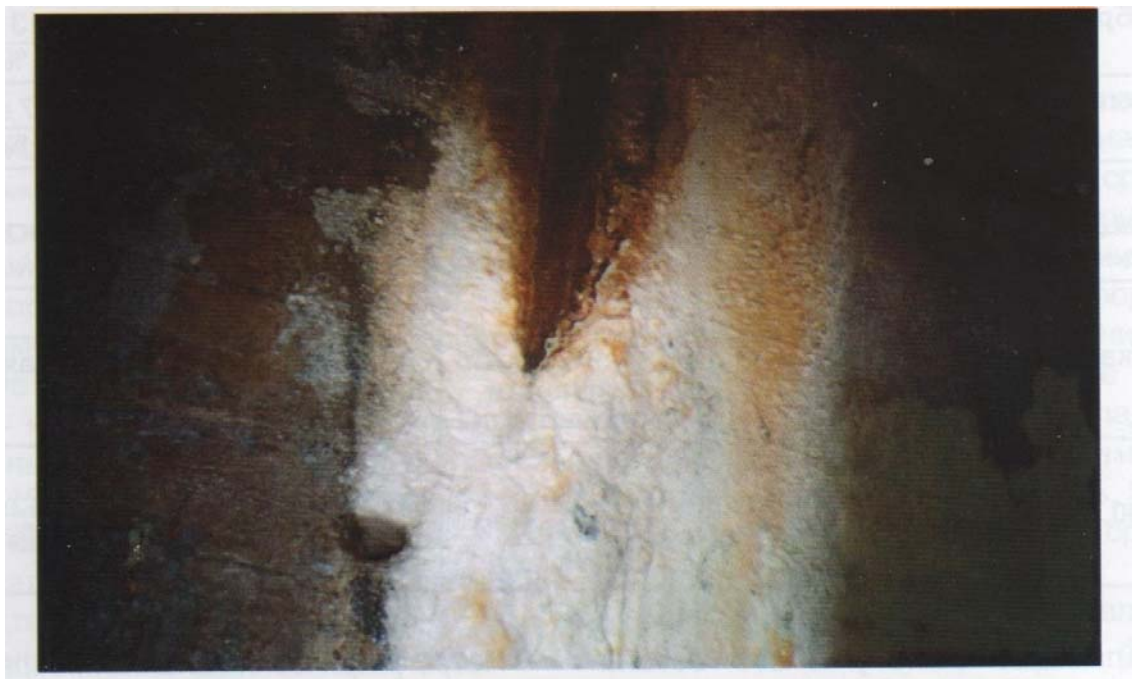
Fig. 3 Calcite sedimentation on an inspection gallery wall.
