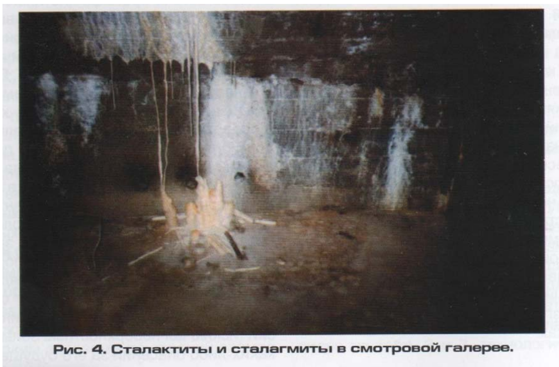
Fig. 4 Stalactites and stalagmites in an inspection gallery.
