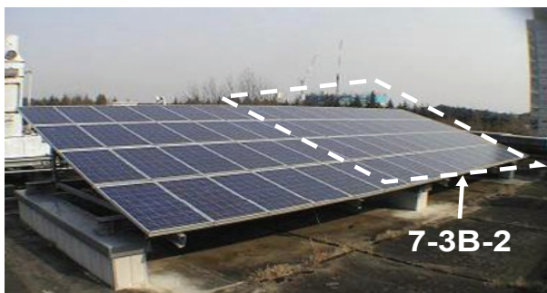
Fig. 1 Appearance of the PV system.
