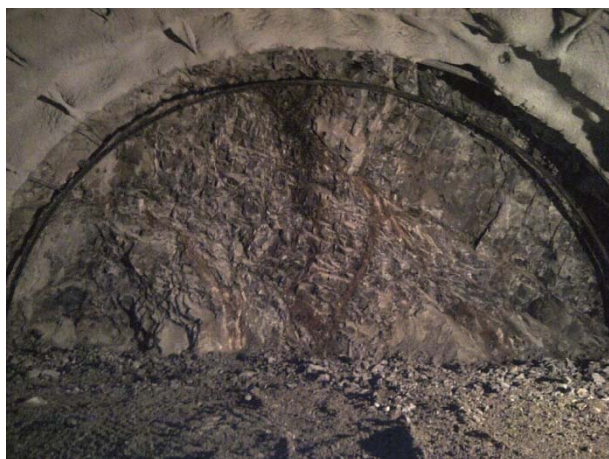
Fig. 6 Gabbro formation during tunneling works of central-west Greece.
