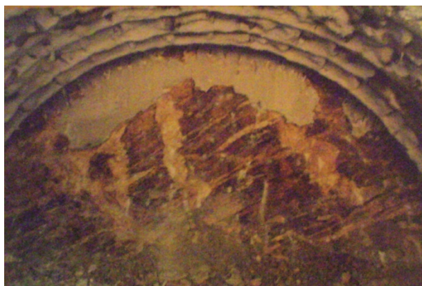
Fig. 4 Weathered and disintegrated rock mass quality at Asprovalta—Strymona's part of Egnatia Highway in Northern Greece.
