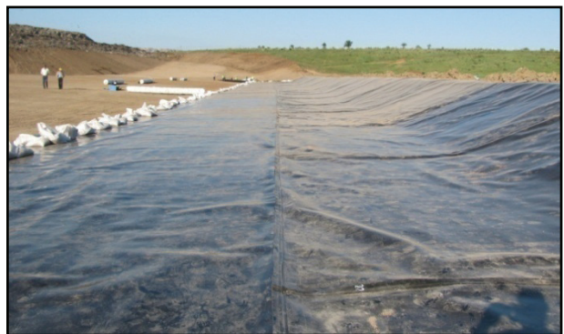
Fig. 11 General impression of the Albota area for the new landfill—Preparation of the base sealing of the new landfill.
