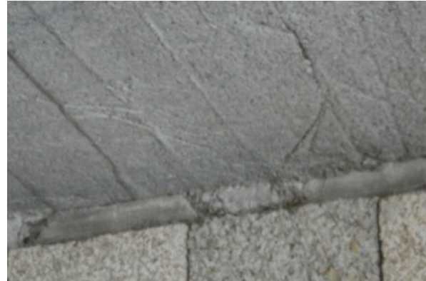
Fig. 5 Interior corner showing wall and roof interface.
