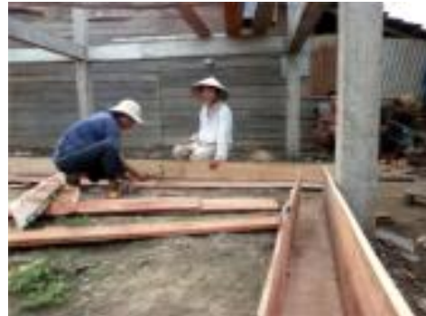
Fig. 5 Executing RC skeleton (left) and installing wooden walls (right) on the site.
