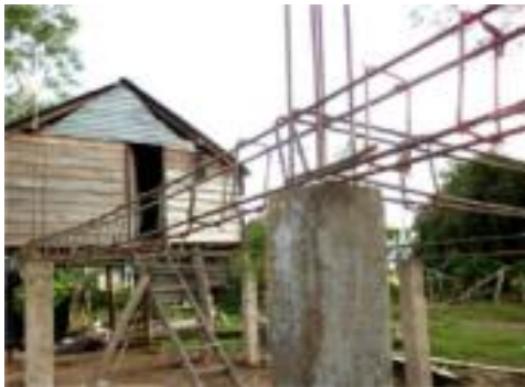
Fig. 5 Executing RC skeleton (left) and installing wooden walls (right) on the site.
