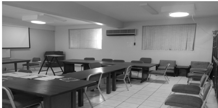
Fig. 2 Experimental room displaying two of the four light pipes under sunny conditions and the light distribution.
